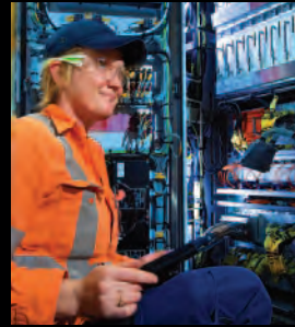
20:10 A maintenance technician tests the vigilance fault, a safety system that sounds an alarm regularly to make sure a train driver is awake.
