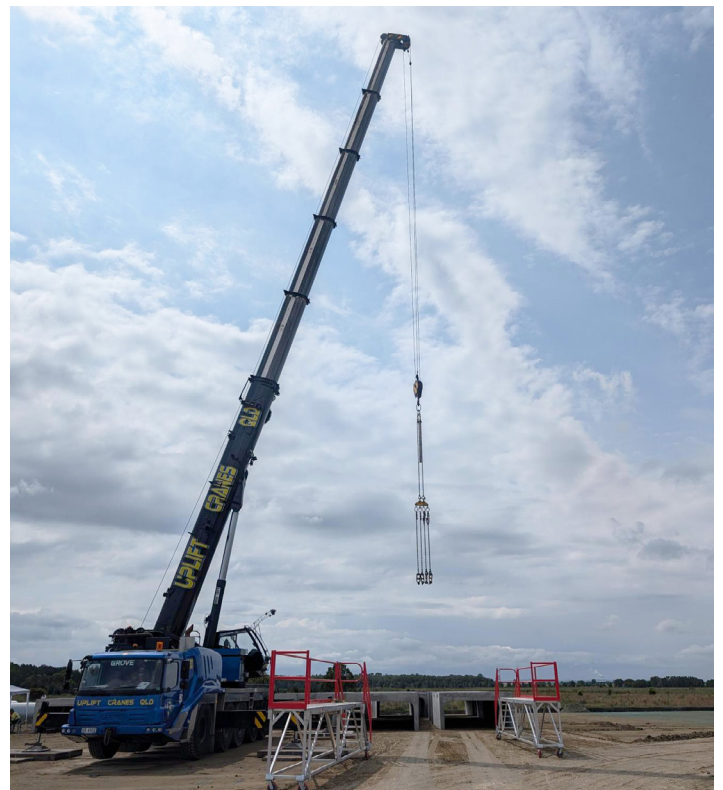
Uplift Cranes on the Ormeau rail facility site
