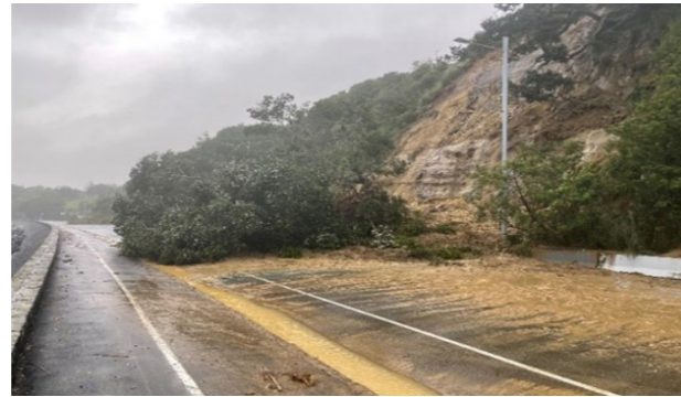
Figure 4: Emergency road closure on Tāmaki Drive in Auckland Jan 2023 – a high impact road with 30k VPD – opened one-way within 48 hours.
